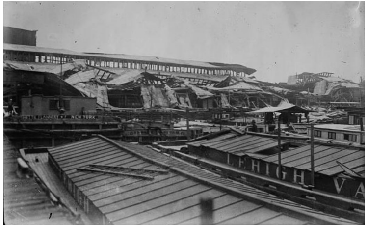
Collapsed warehouses on Jersey City's Black Tom Island rail terminal. The terminal served as a vital link in the shipment of munitions from American factories to the Entente powers of Europe. During the early morning hours of July 31, 1916, watchmen discovered fires had been set amongst ammunition laden railcars. The ensuing explosion caused skyscrapers in Manhattan to sway, smashed windows dozens of miles away, and was heard as far away as Philadelphia.
